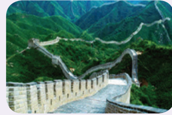
The Great Wall of China
