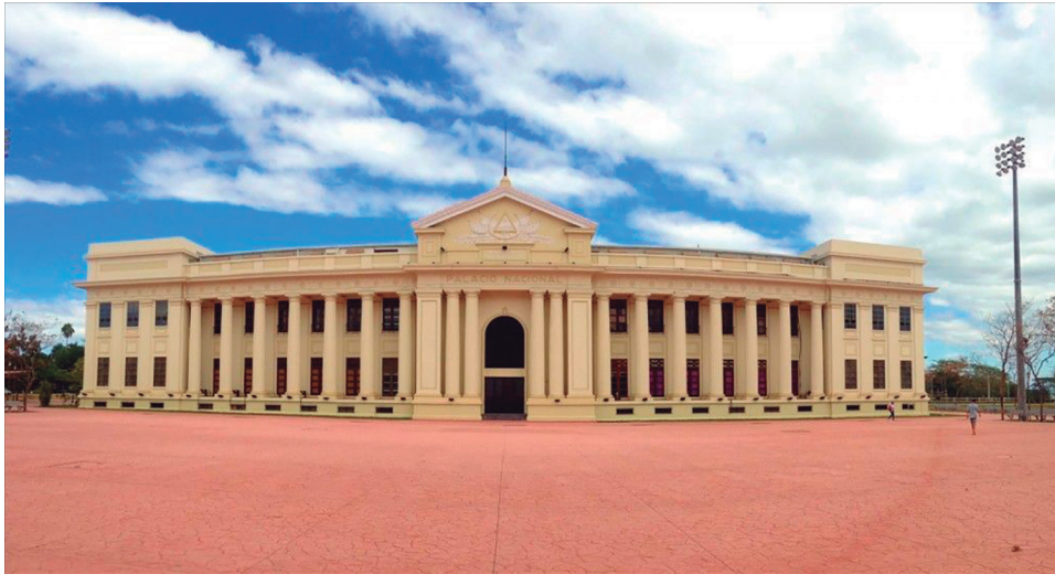
Fachada principal PNC
